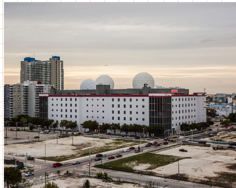
The Network Access Point of the Americas in downtown Miami, Photo credit: David Greer, Used with permission.
